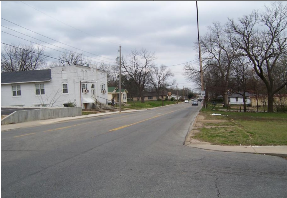
View looking Easterly along Washington Ave.
