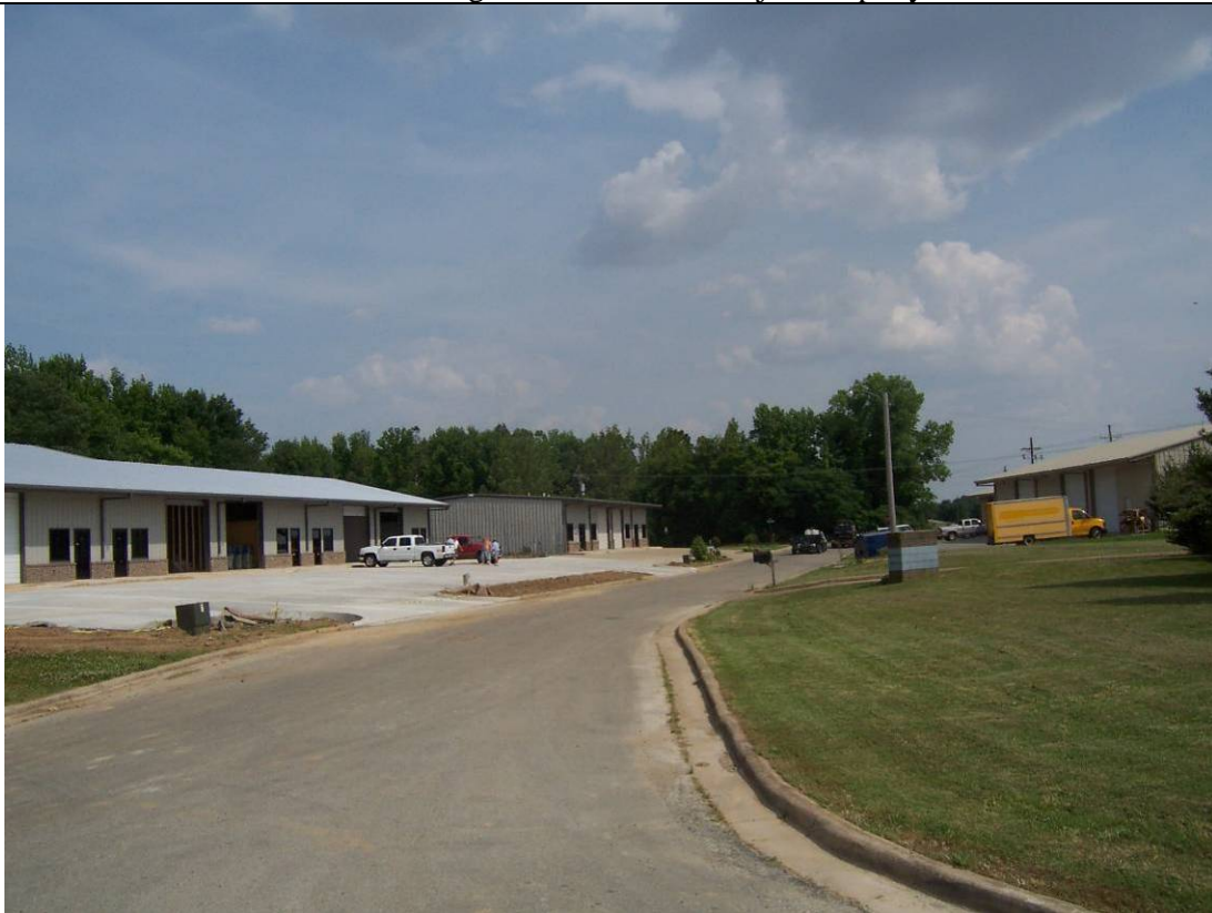
View Looking Southeast toward Subject Property
