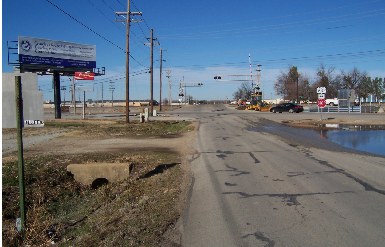
View looking north along Industrial Dr.
