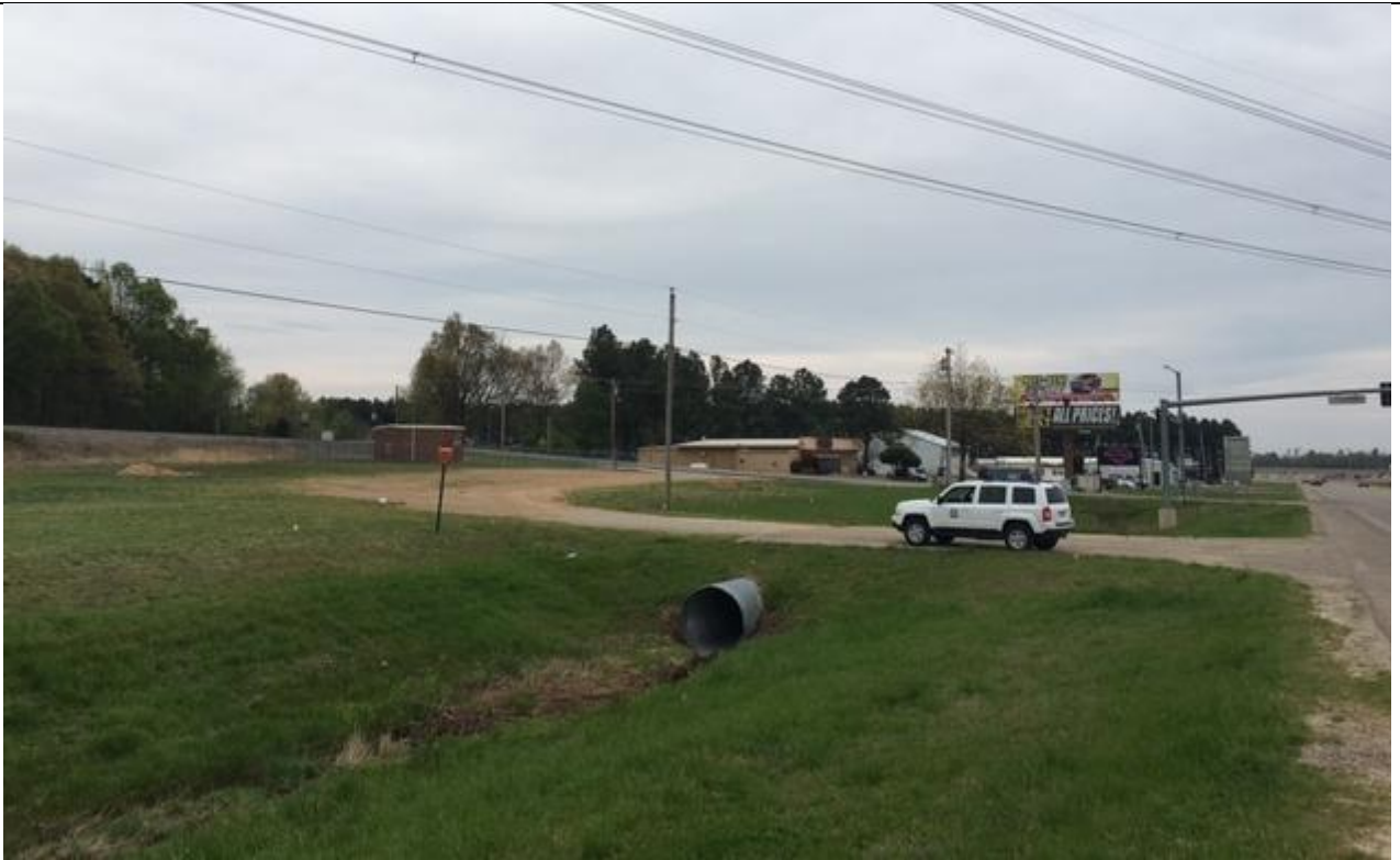
View looking South Toward Site
