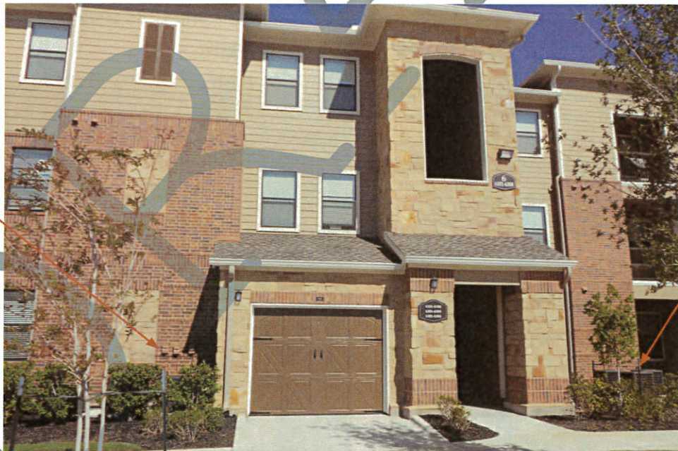
Painted to match building material.
