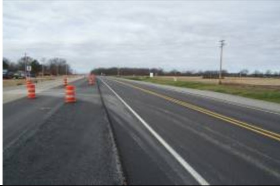
View Looking West along Hwy 49
