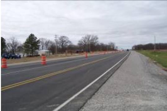
View Looking West along Hwy 49
