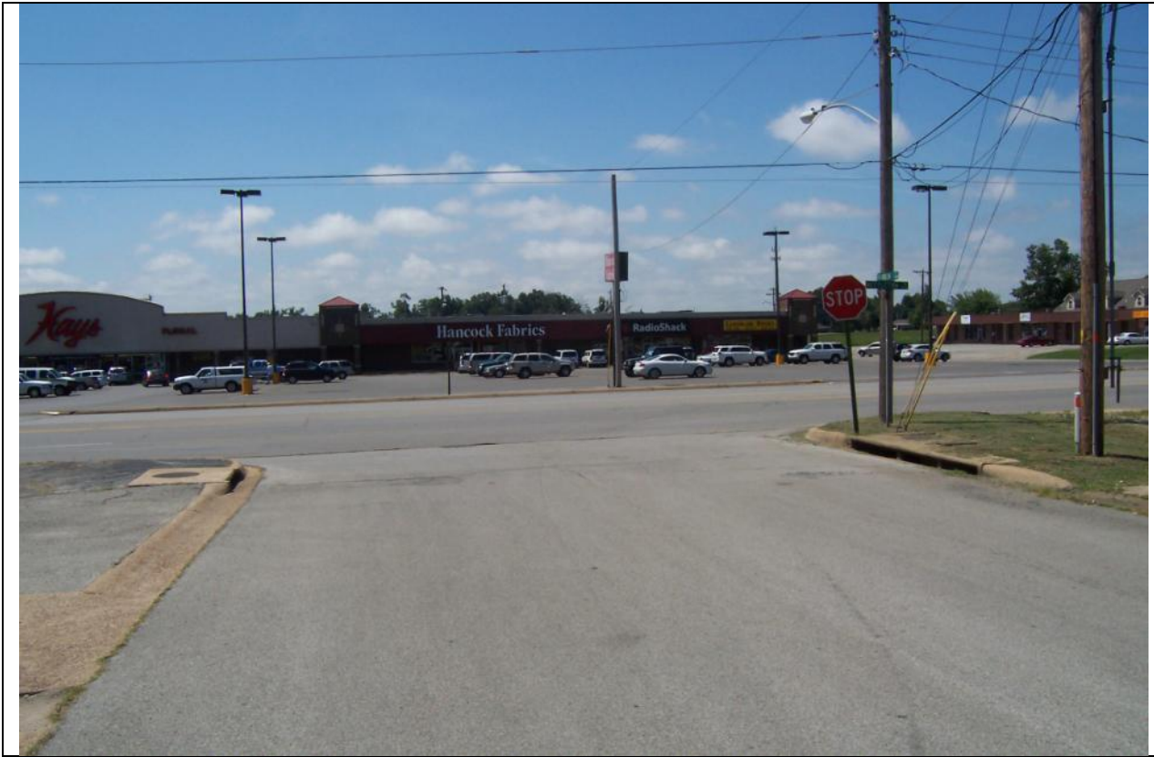
View looking south of the site
