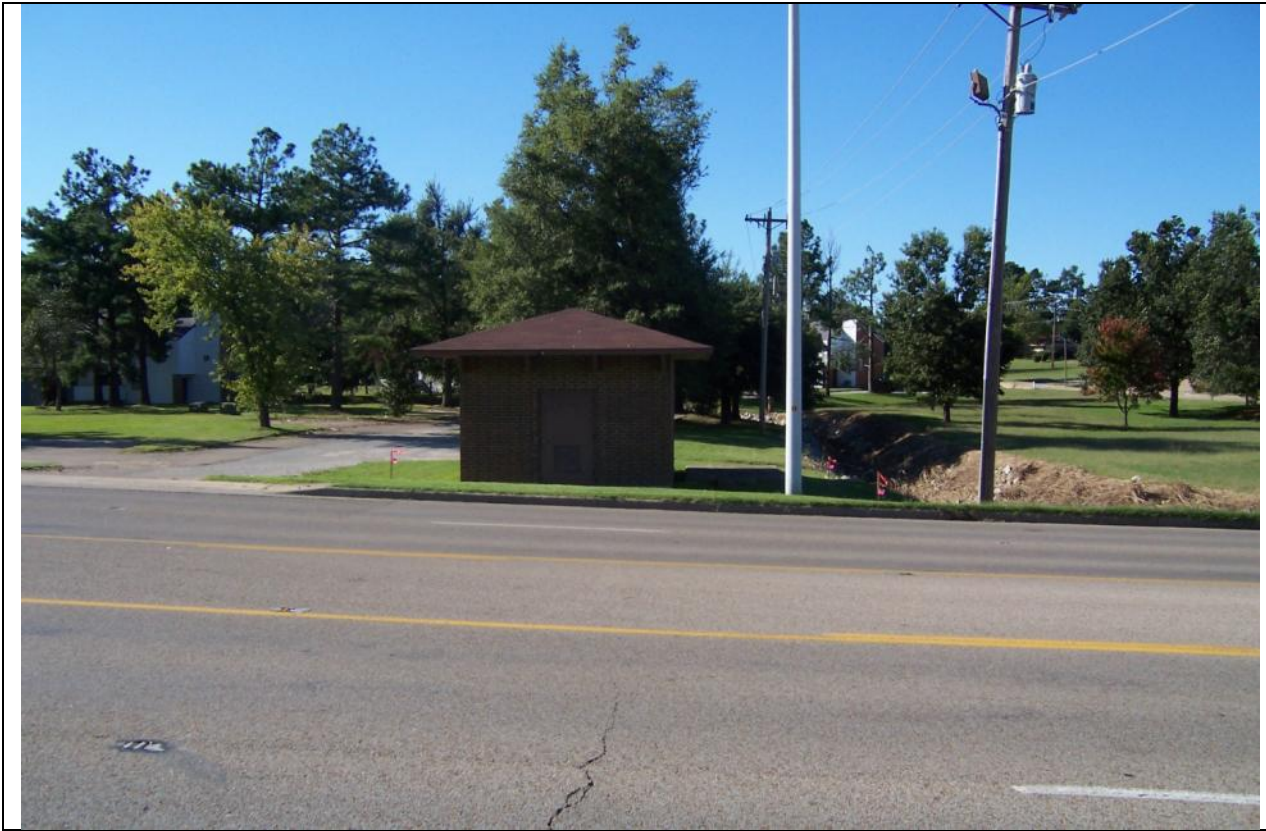
View Looking Northeast at the site
