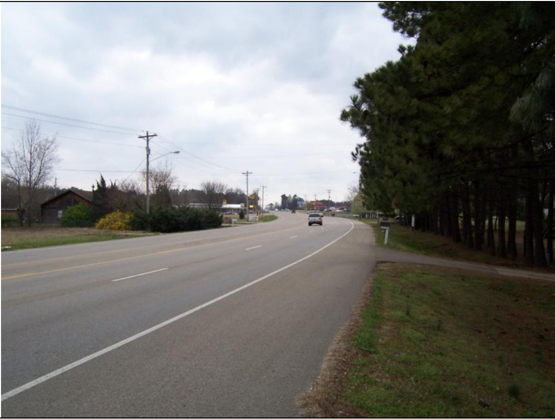
View looking southwest
