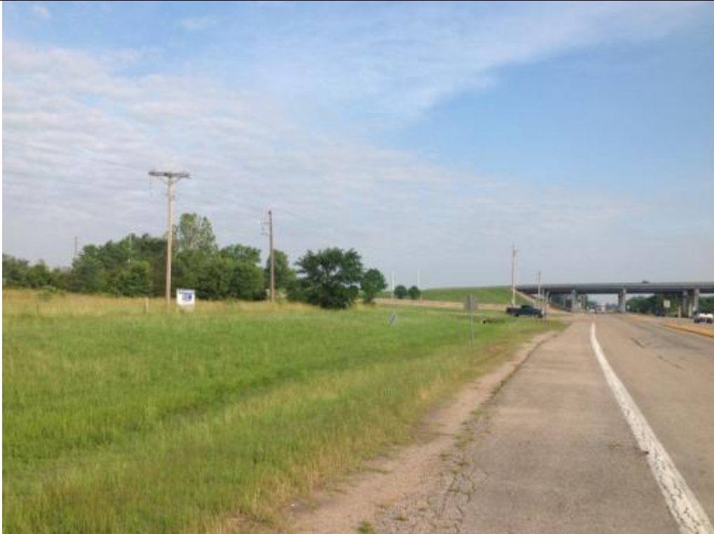
View looking North towards I-63 / I-463 Interchange
