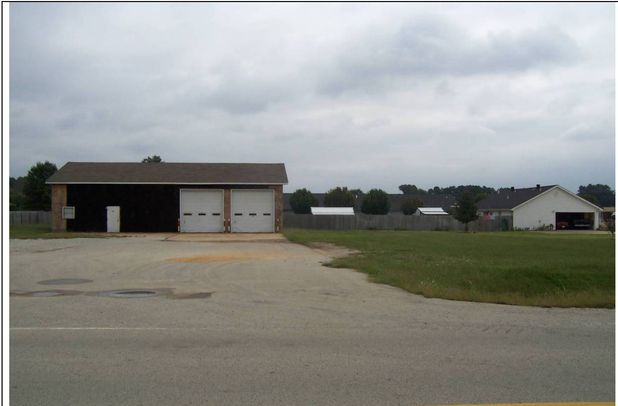
View Looking East from the Subject Property
