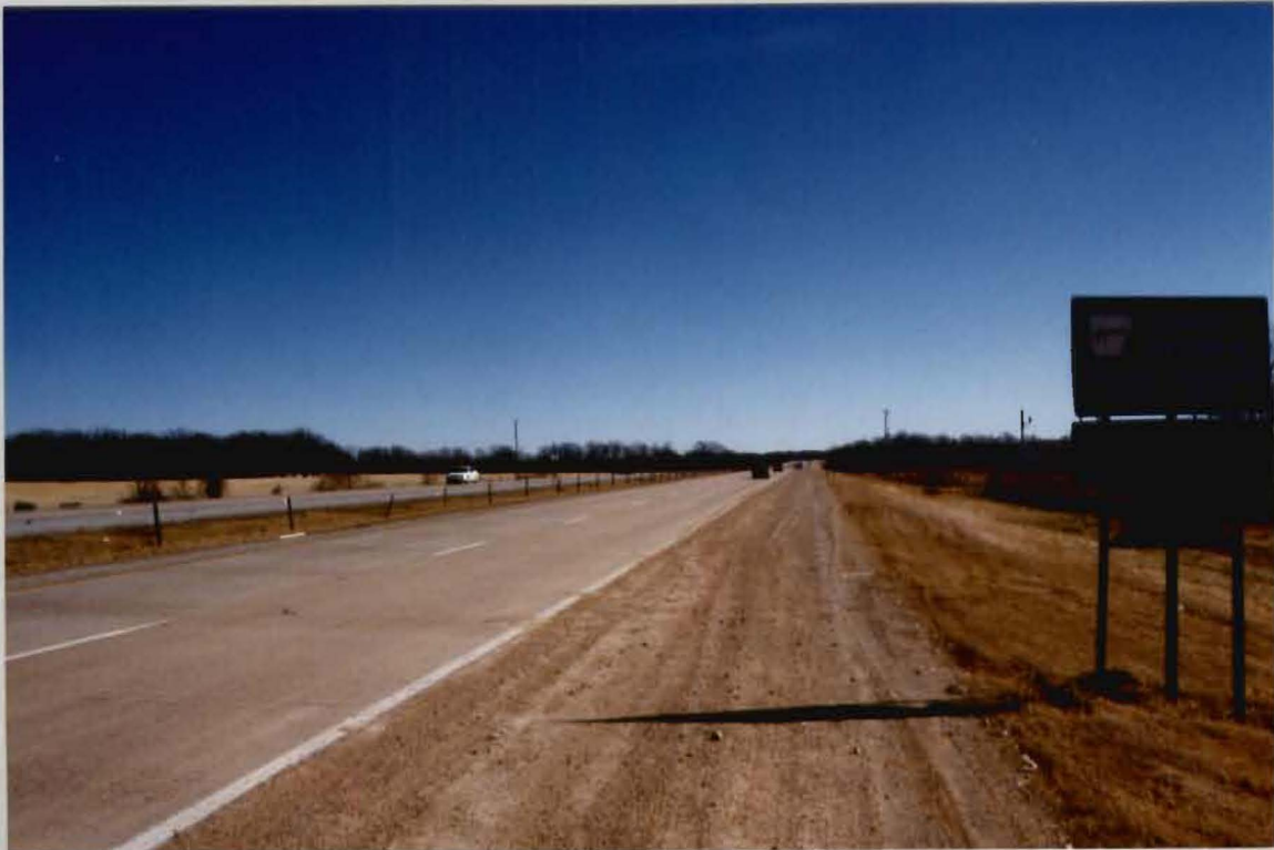
HIGHWAY VIEW - SOUTH/EAST
