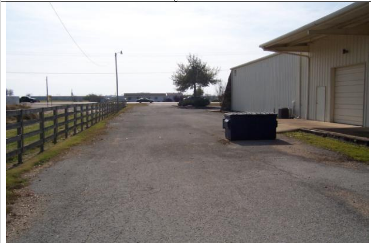
View looking south along Highland Dr.
