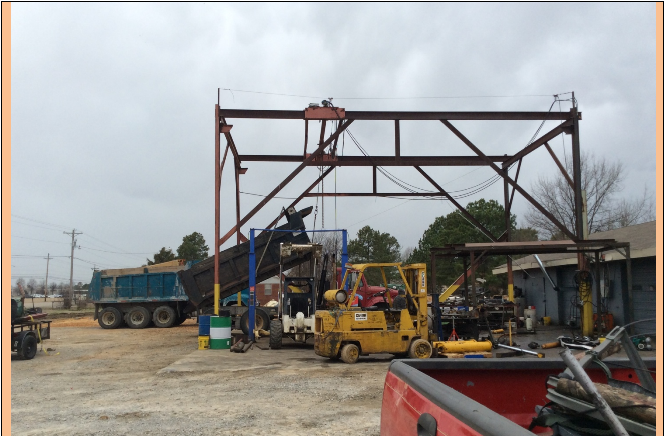
View looking West on Site
