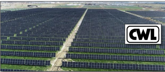
CWL Solar Park – 98 acres in the Craighead Technology Park – 13.25 Megawatt capacity
