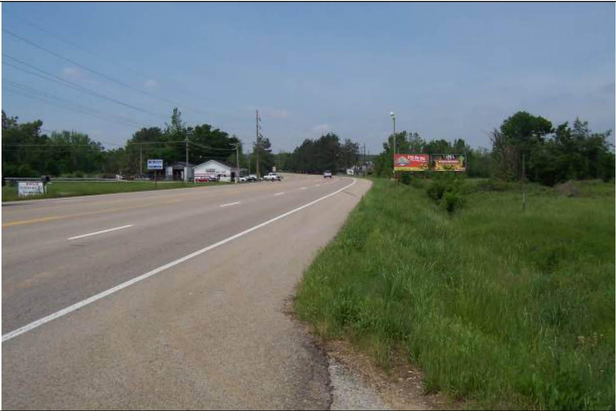
View looking West Along Highway 49 N
