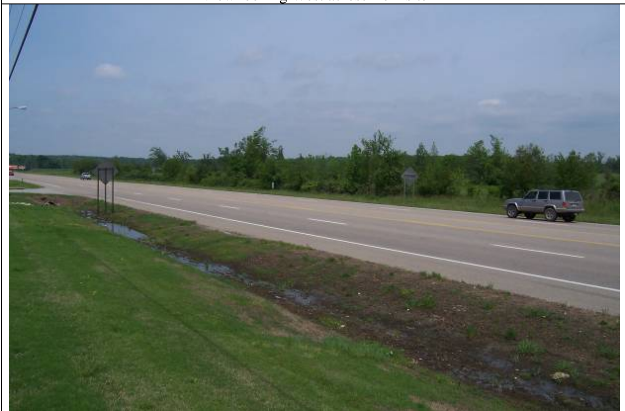
View looking Northwest along Hwy. 49 N. towards site
