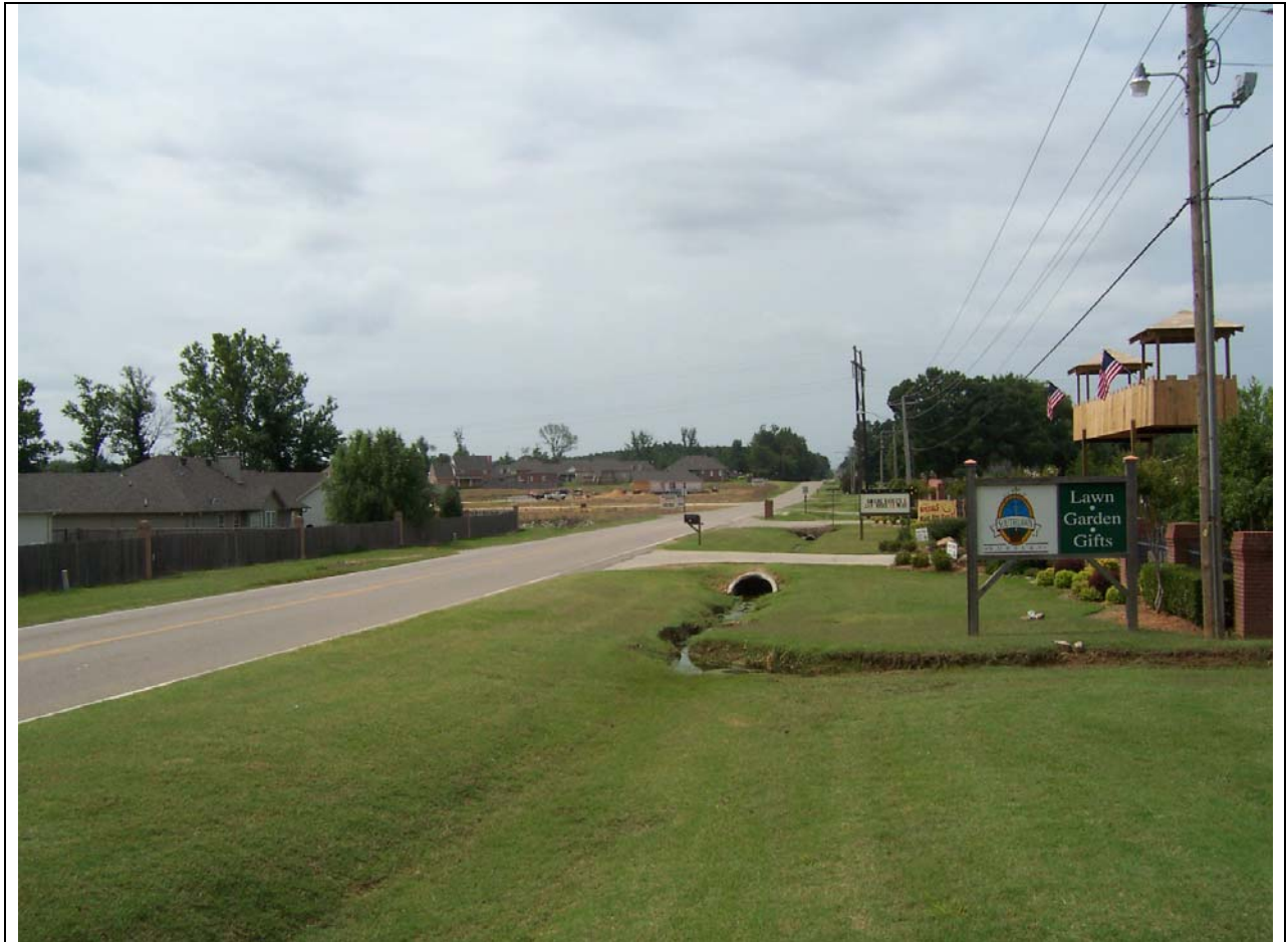
View looking south along S. Culberhouse Rd.
