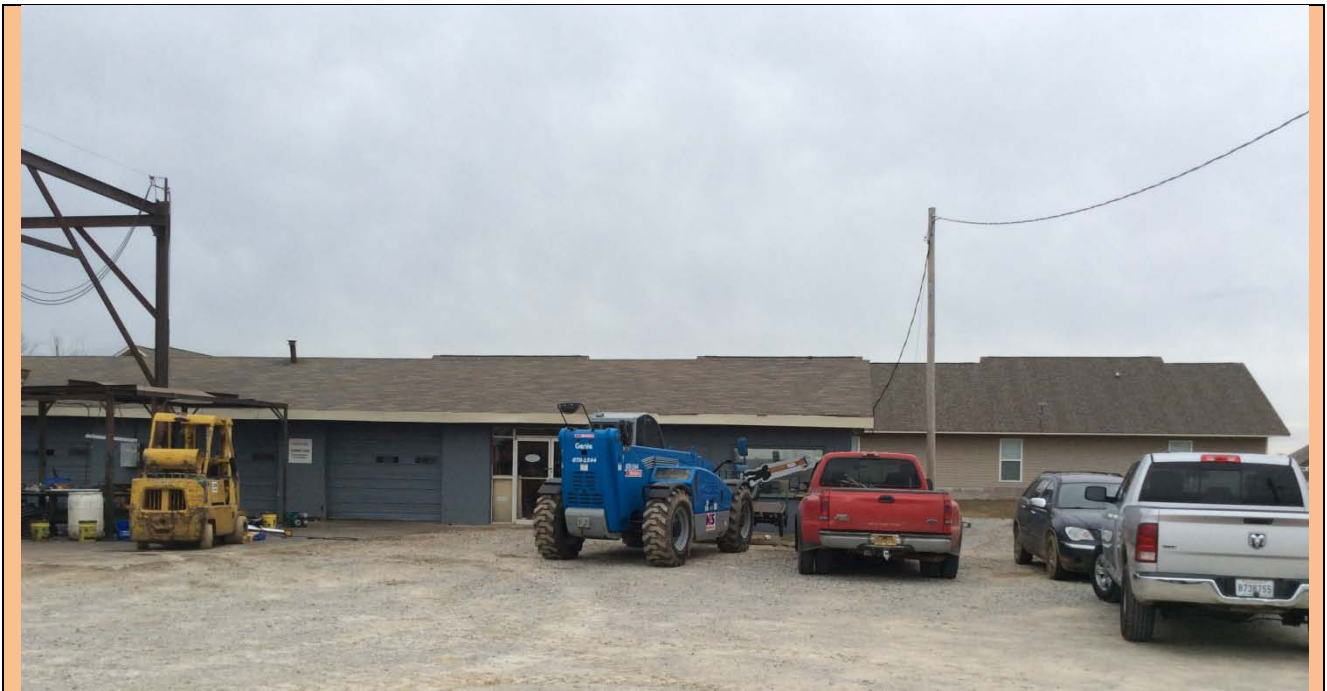
View looking North
