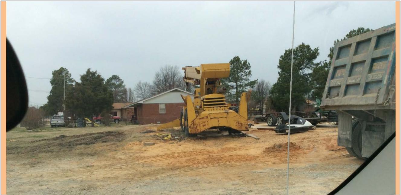
View looking West from Site
