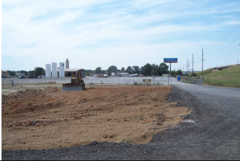
View looking west along Parker Rd.
