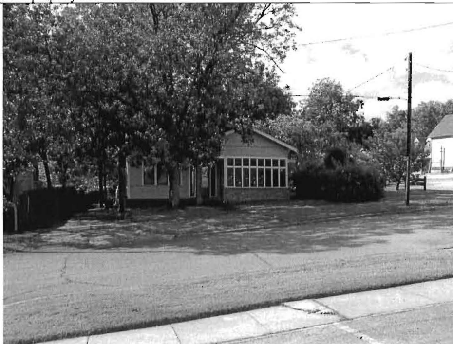
Eastward view of the subject property
