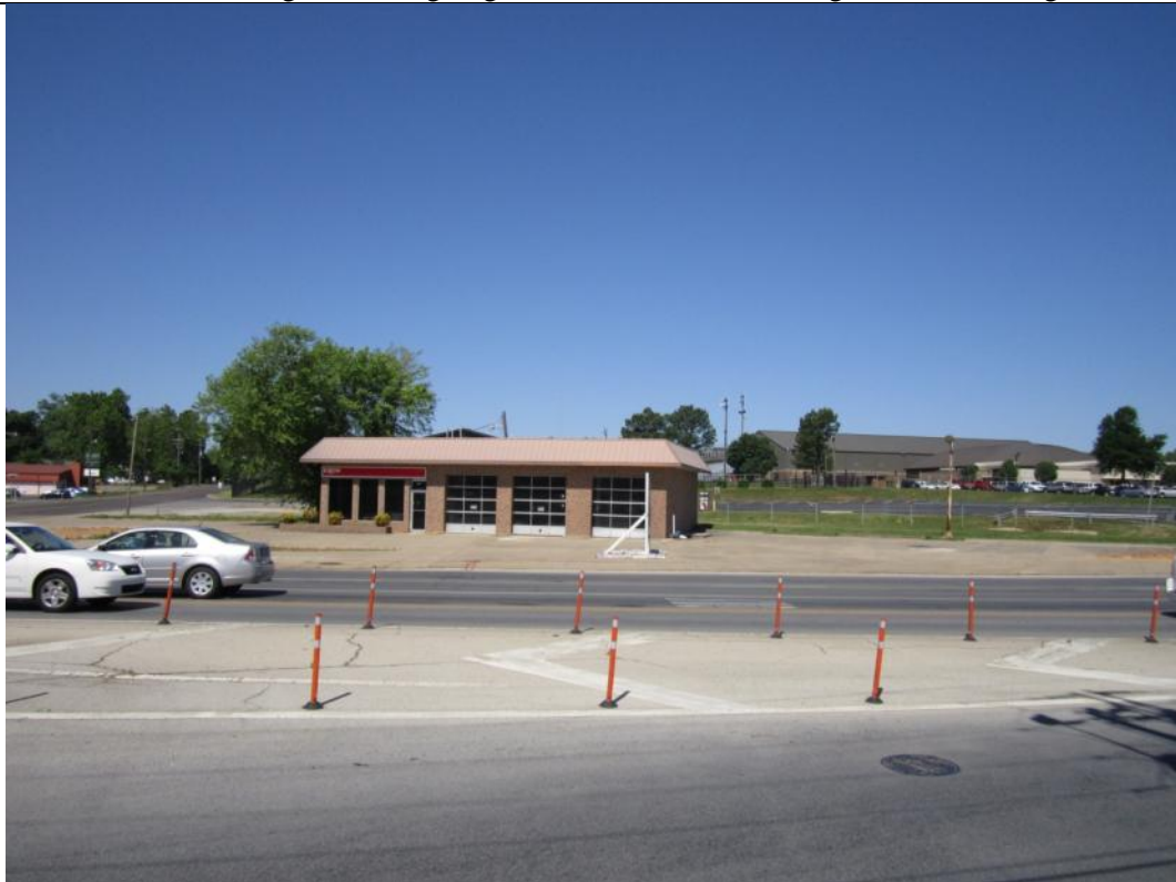
View looking west towards subject property
