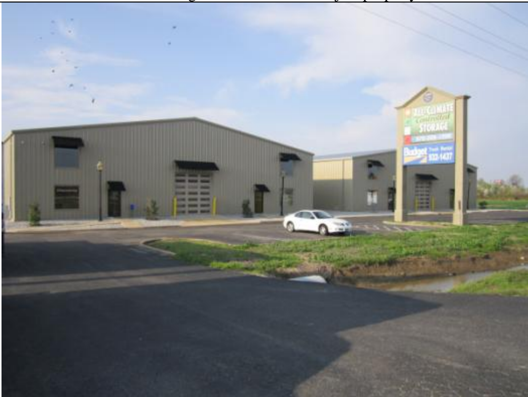
View looking southwest toward 3309 E. Parker Rd which is located west of subject property.
