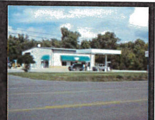
Fig. 5: Example Rural Development Type-Service Commercial-Fueling Station
