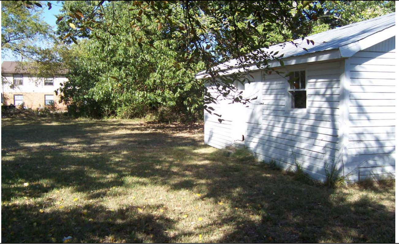
View looking north of the rear yard.
