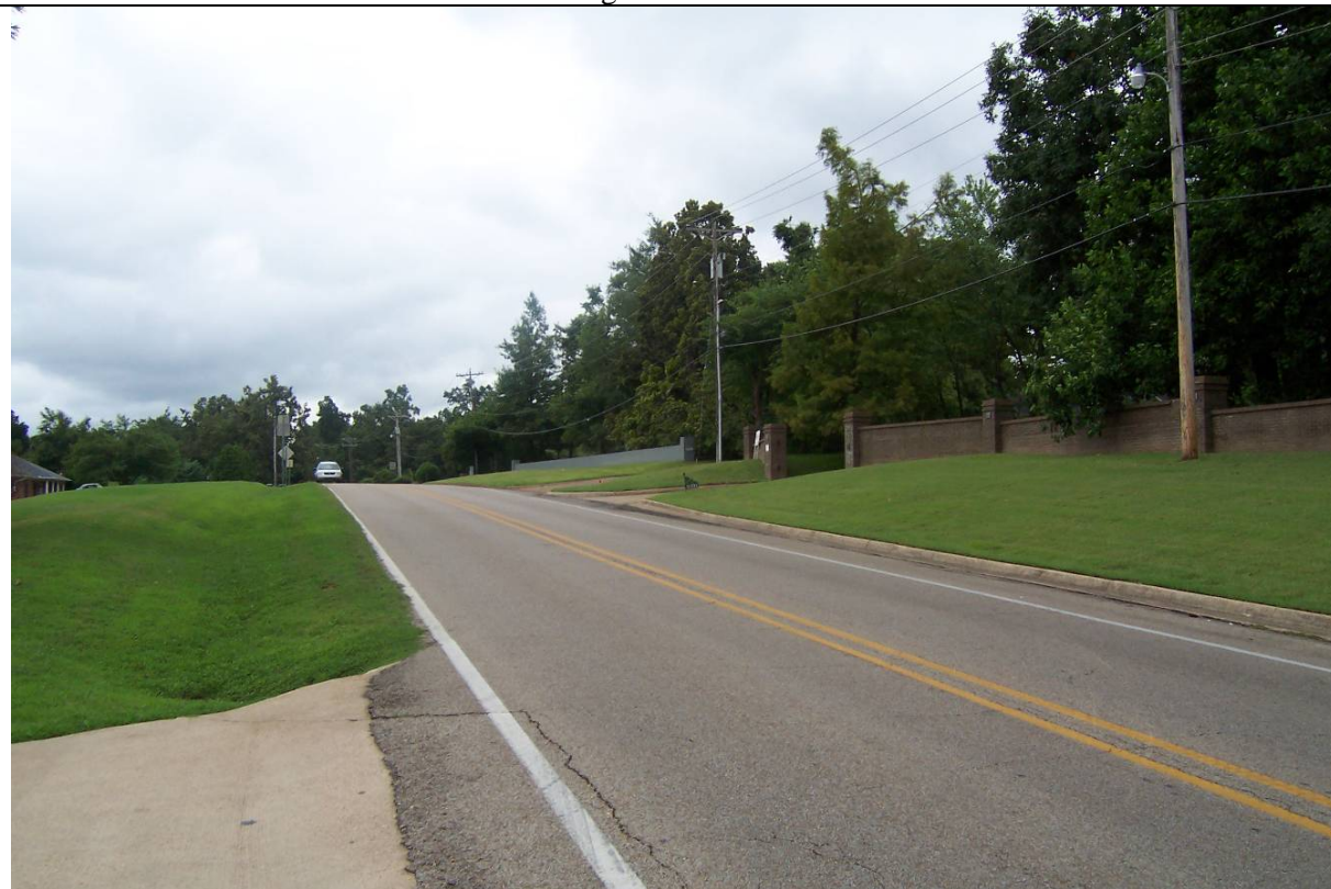
View looking South on Harrisburg
