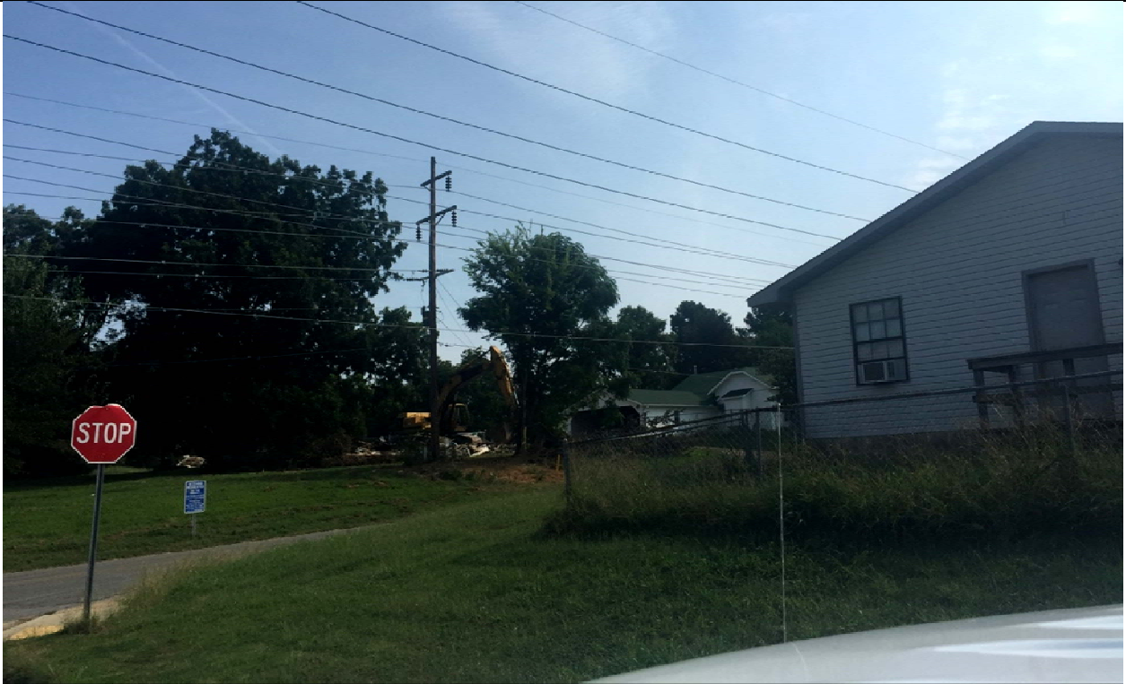
View from Calion St. looking towards site
