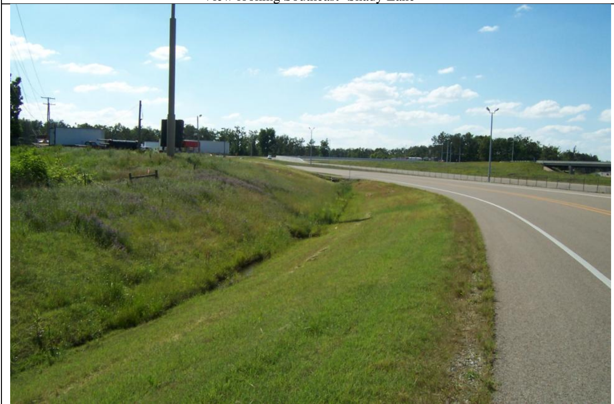
View looking Northwest (W. Parker Rd.)
