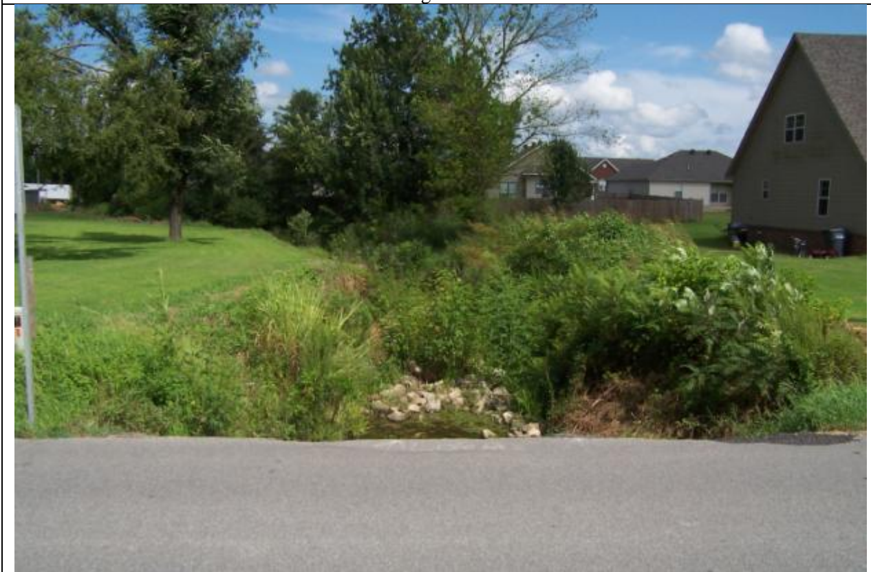
View looking east along ditch (south property line).
