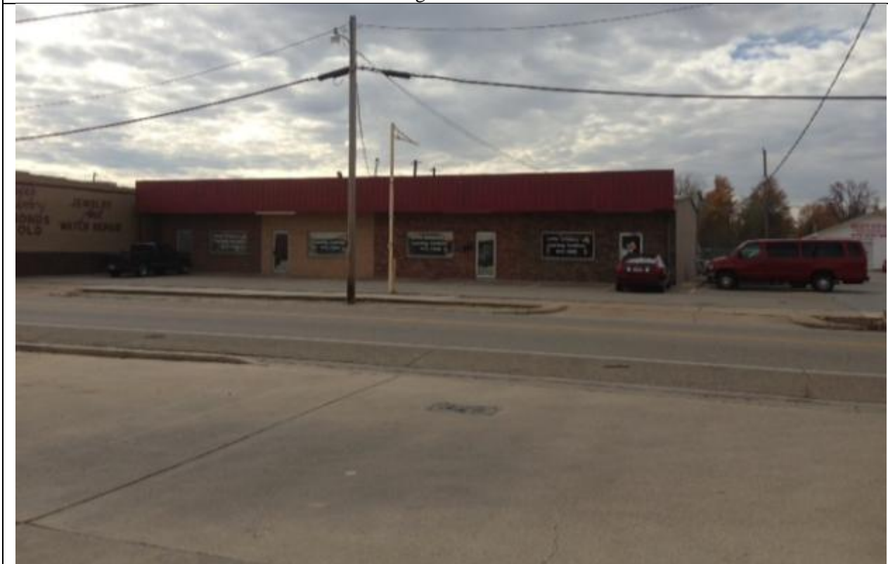
View looking South at existing building
