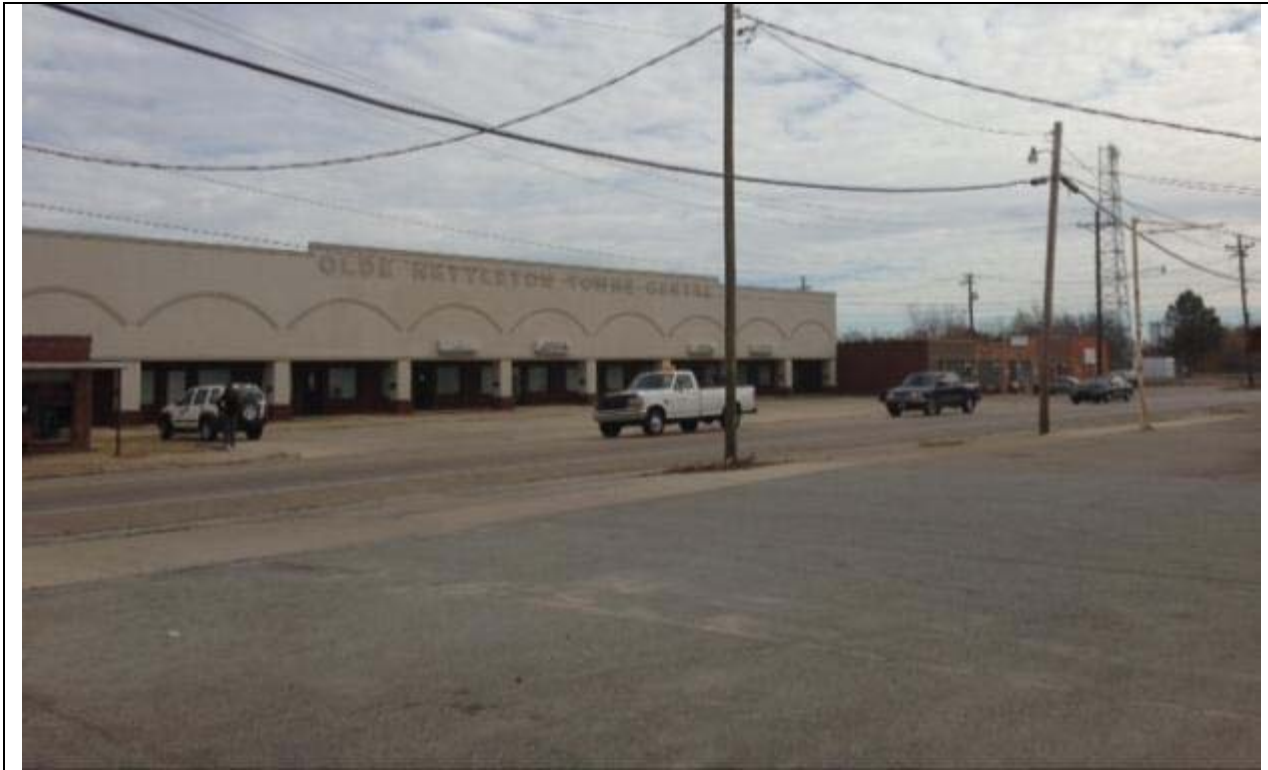
View looking Northeast from Site
