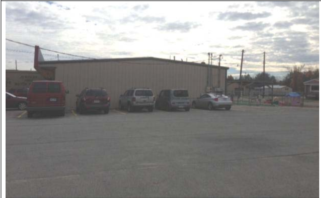
View looking east at building structure
