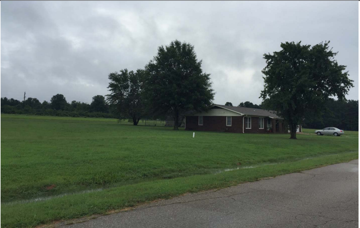
View looking Northeast along Jonathan toward property location
