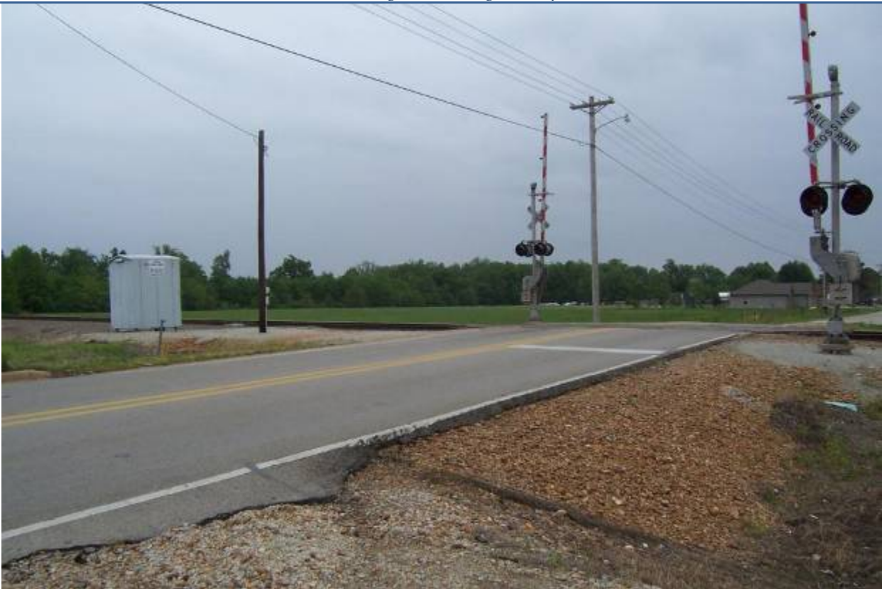
View looking Northeast towards site
