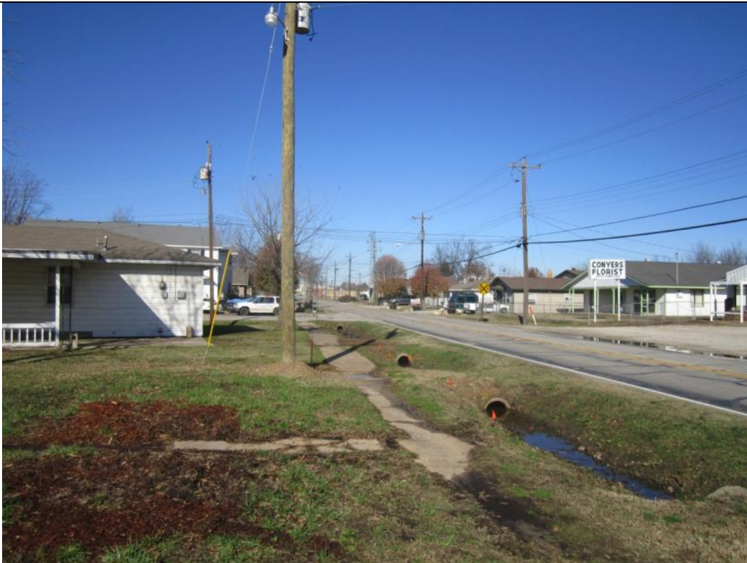
View looking Northwest of along E. Nettleton Ave.
