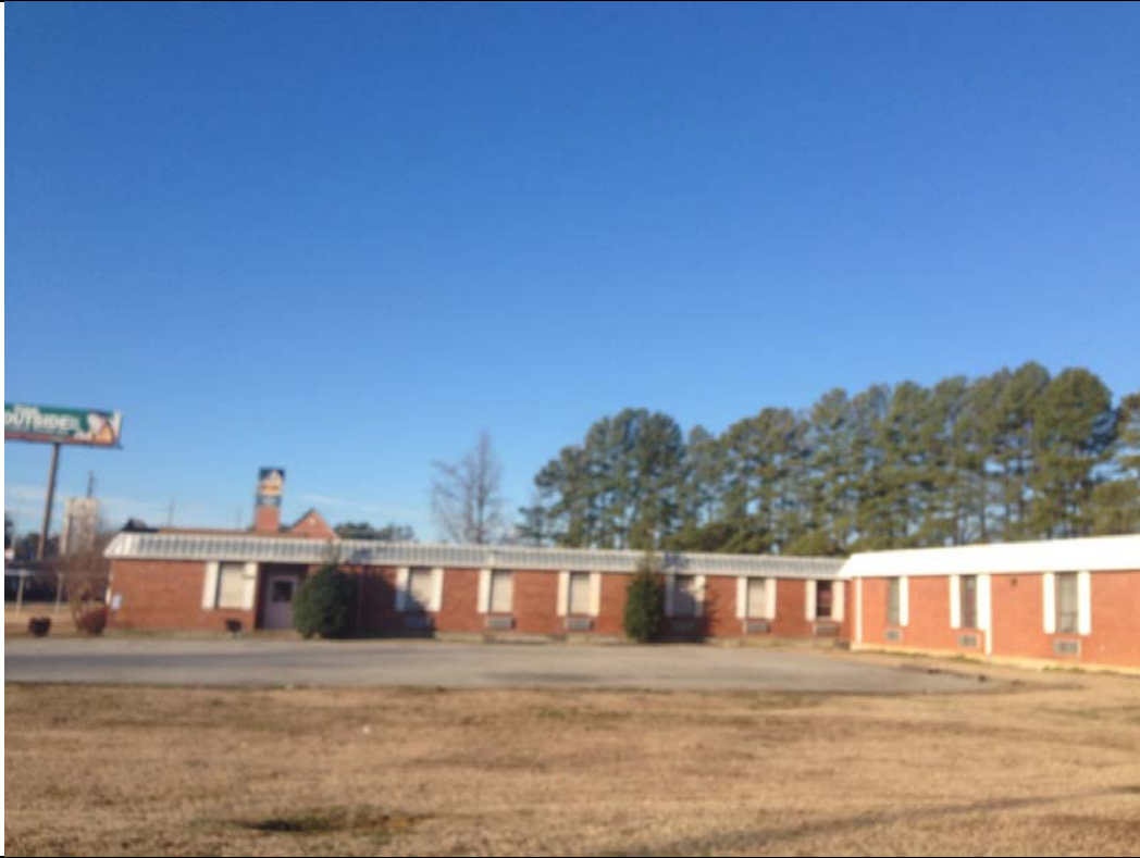
View looking South towards facility
