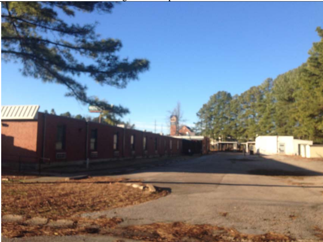
View looking south towards the service drive parking lot and entrance
