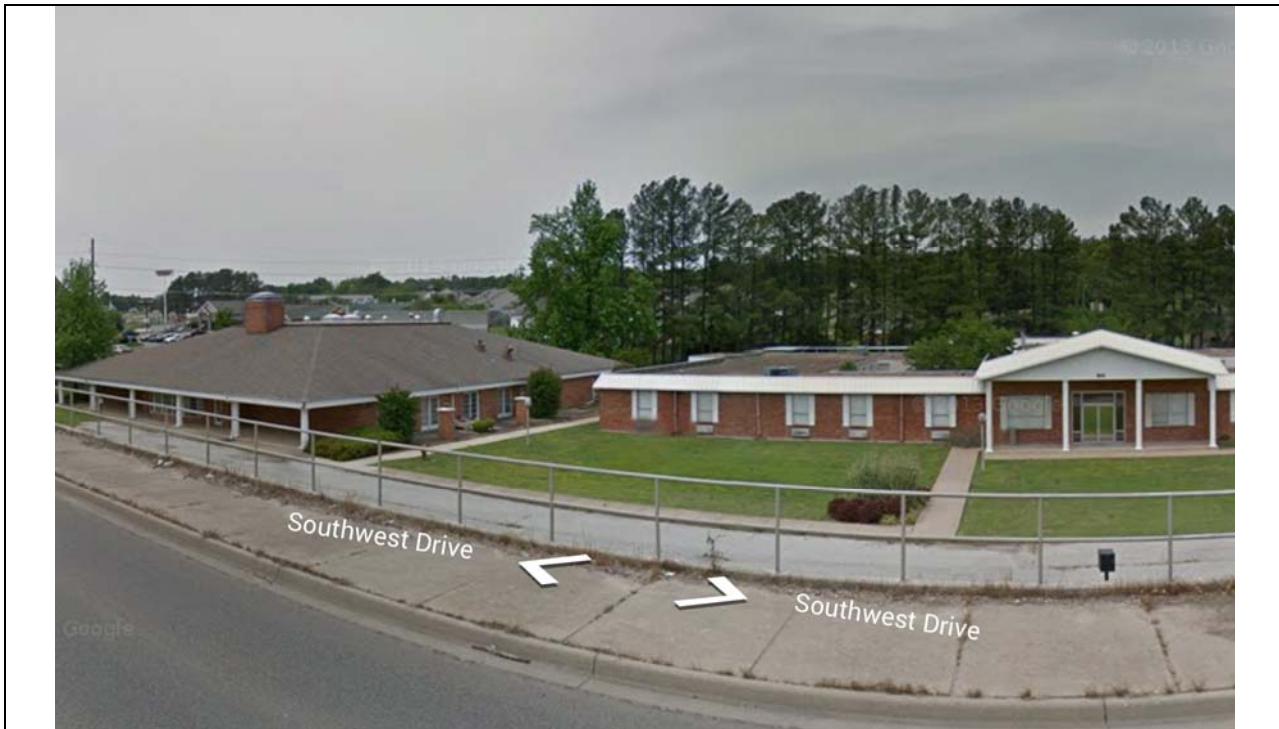
Street View Looking West towards Site
