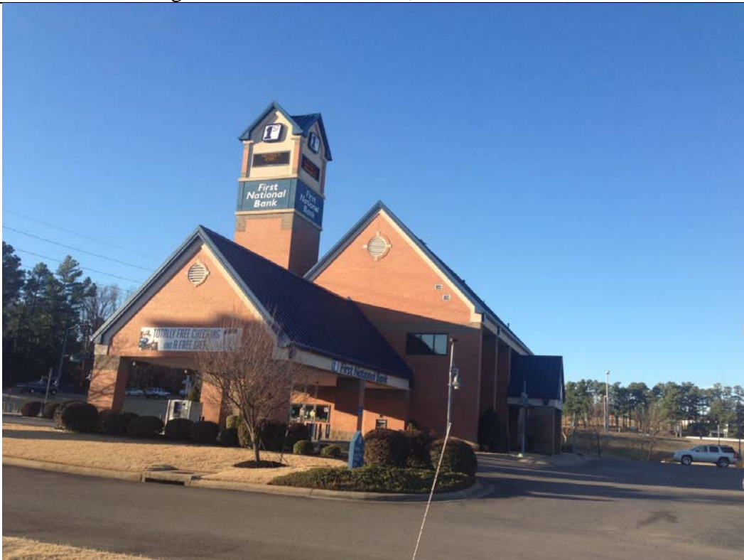
View looking South towards Commercial
