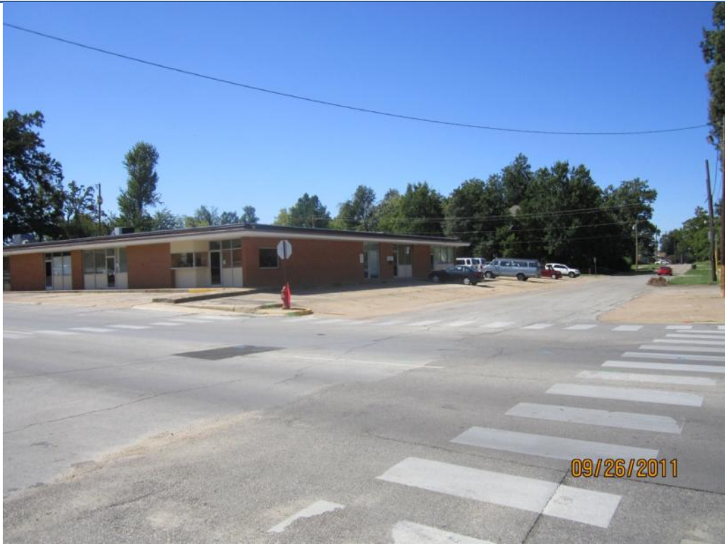
View looking West of church property.
