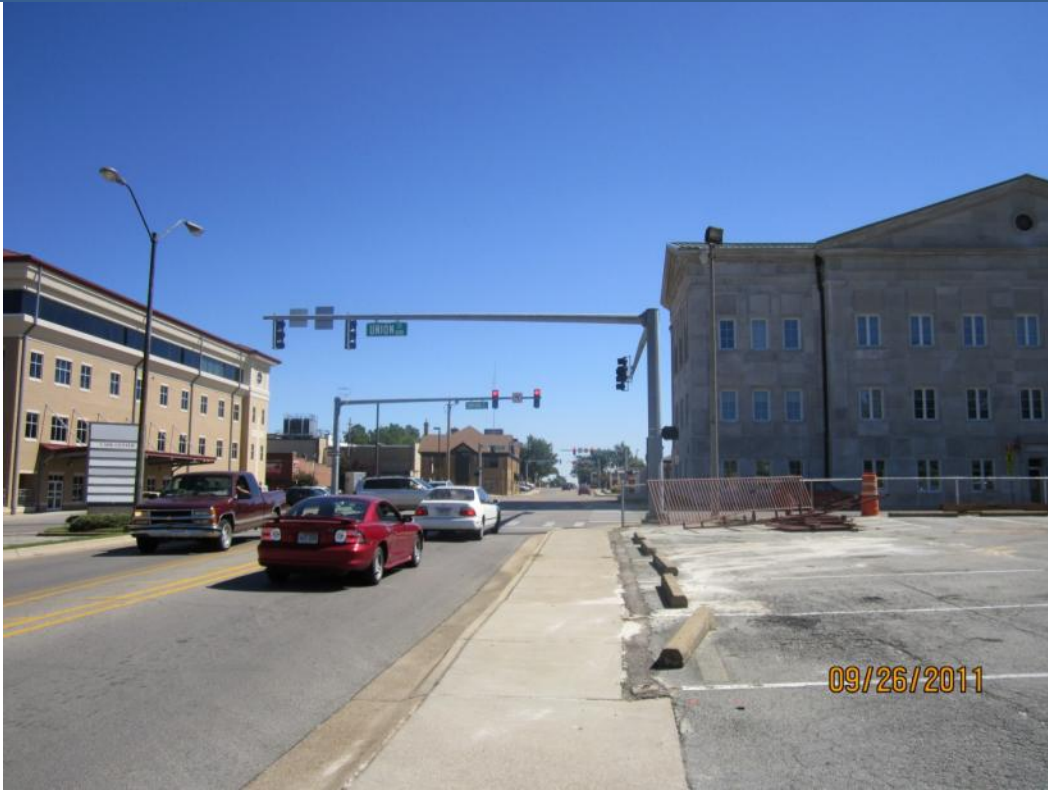
View looking East along Matthews Ave.
