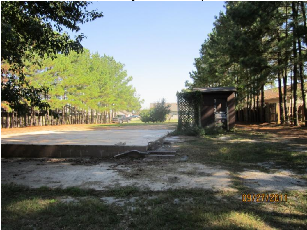
View looking East from the rear yard.
