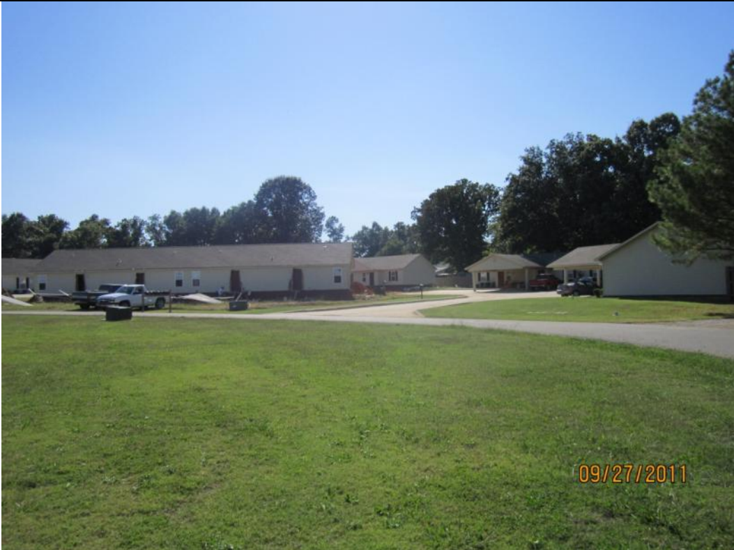
View looking South from the site.
