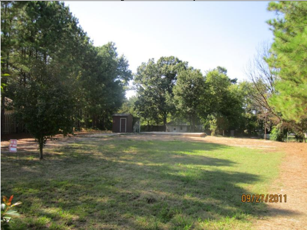
View looking West of demolished Single Family Home foundation and storage buildings.
