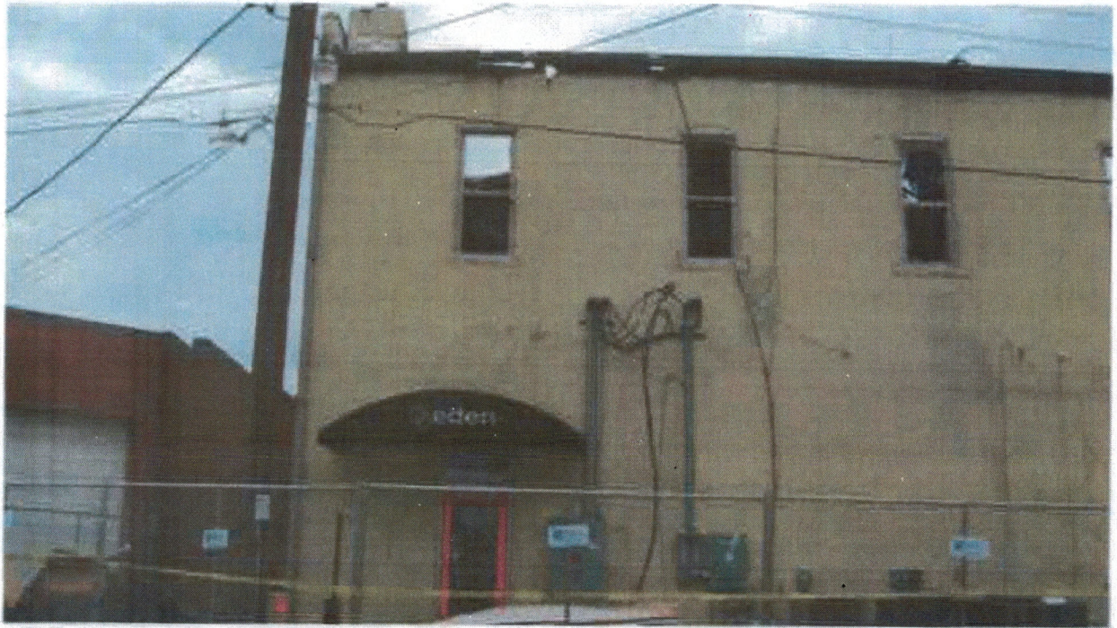
Photo 41 - West face of building.
