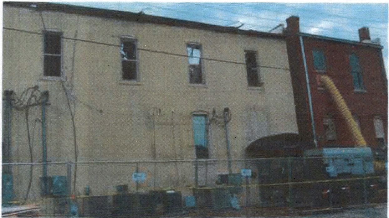
Photo 42 - West face of building.
