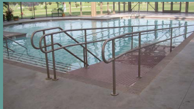
Therapy pools can include accessible ramps for entry for wheelchair users and individuals with mobility difficulties.
