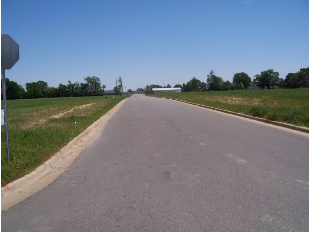
View of the site looking to the east
