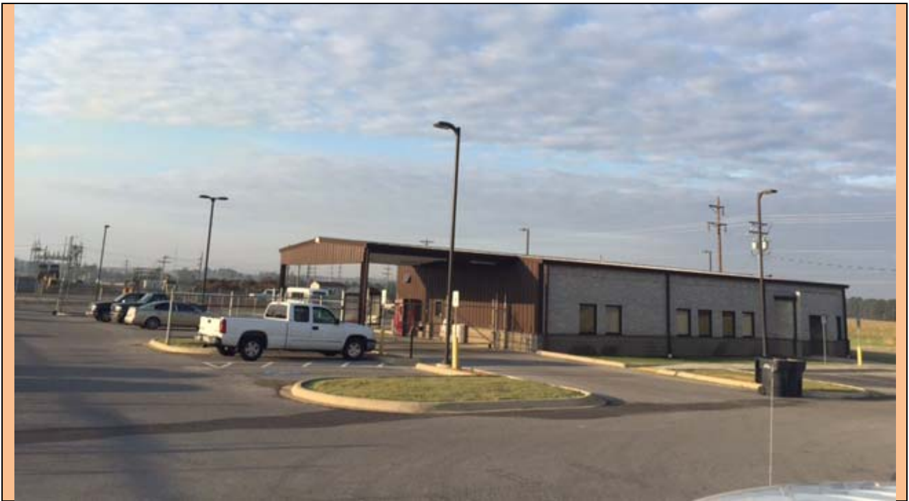
View looking South Towards Jets Facility
