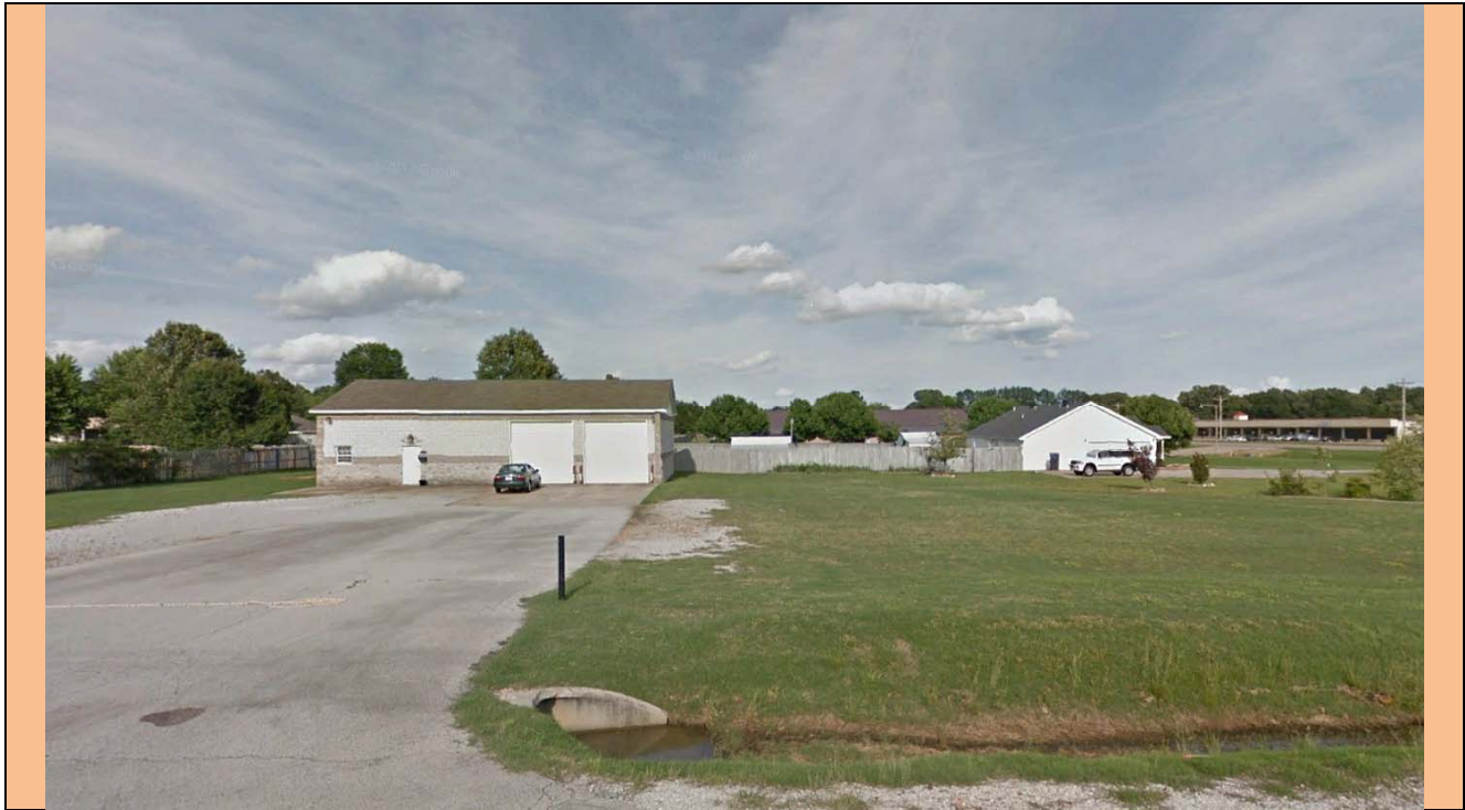
View looking East
