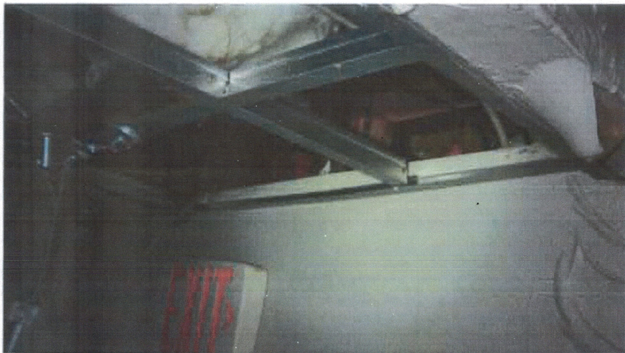
Photo 8- Basement ceiling. Brick wall is visible between joist above suspended ceiling.
