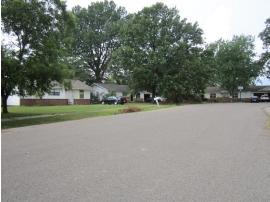
View looking northwest toward subject property fronting Fair Cove.
