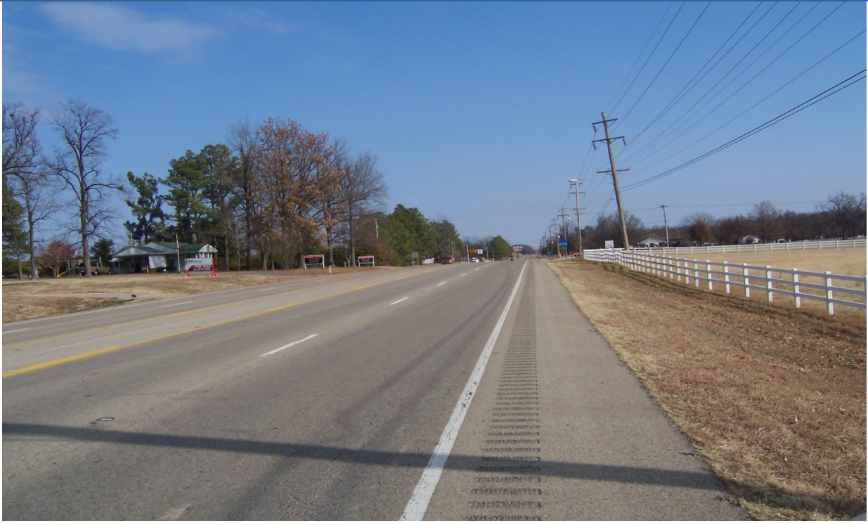
View looking East along Johnson Ave.
