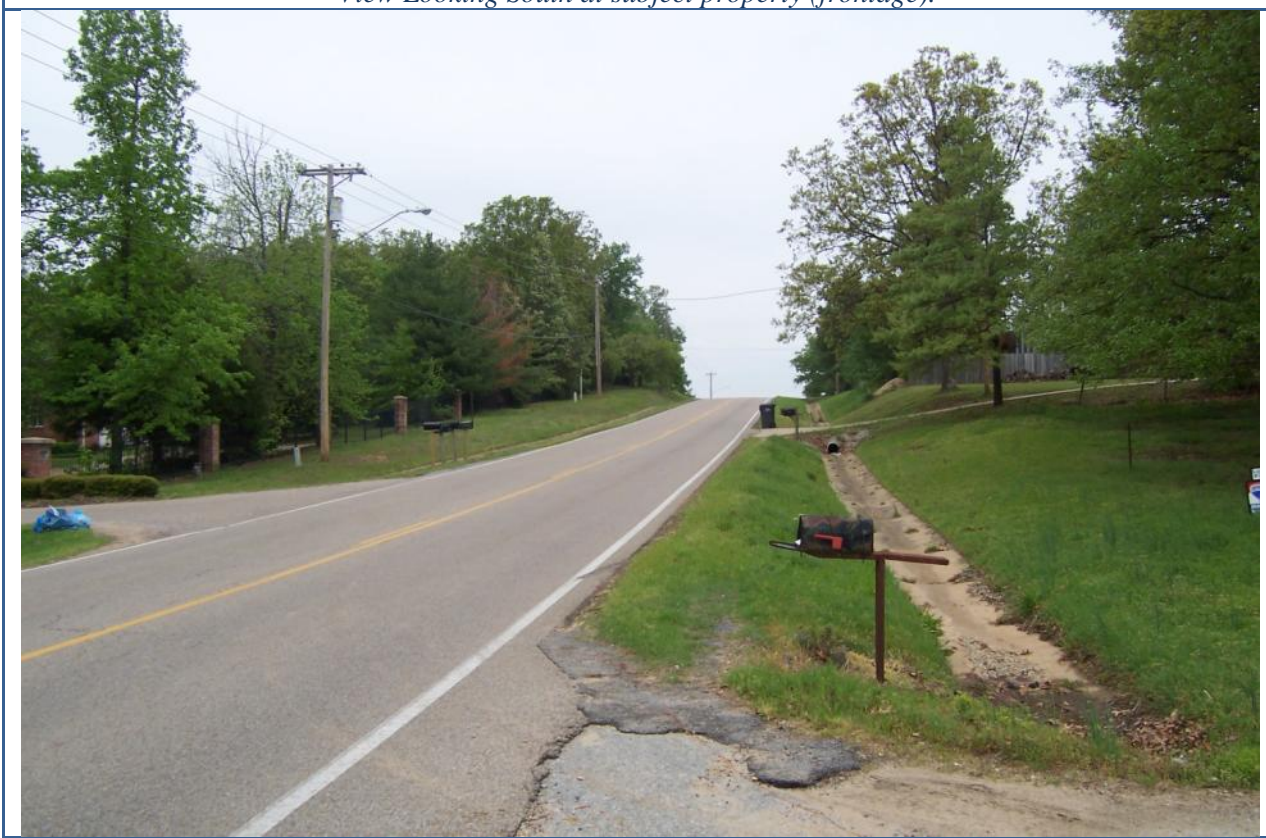
View Looking North at subject property (frontage).
