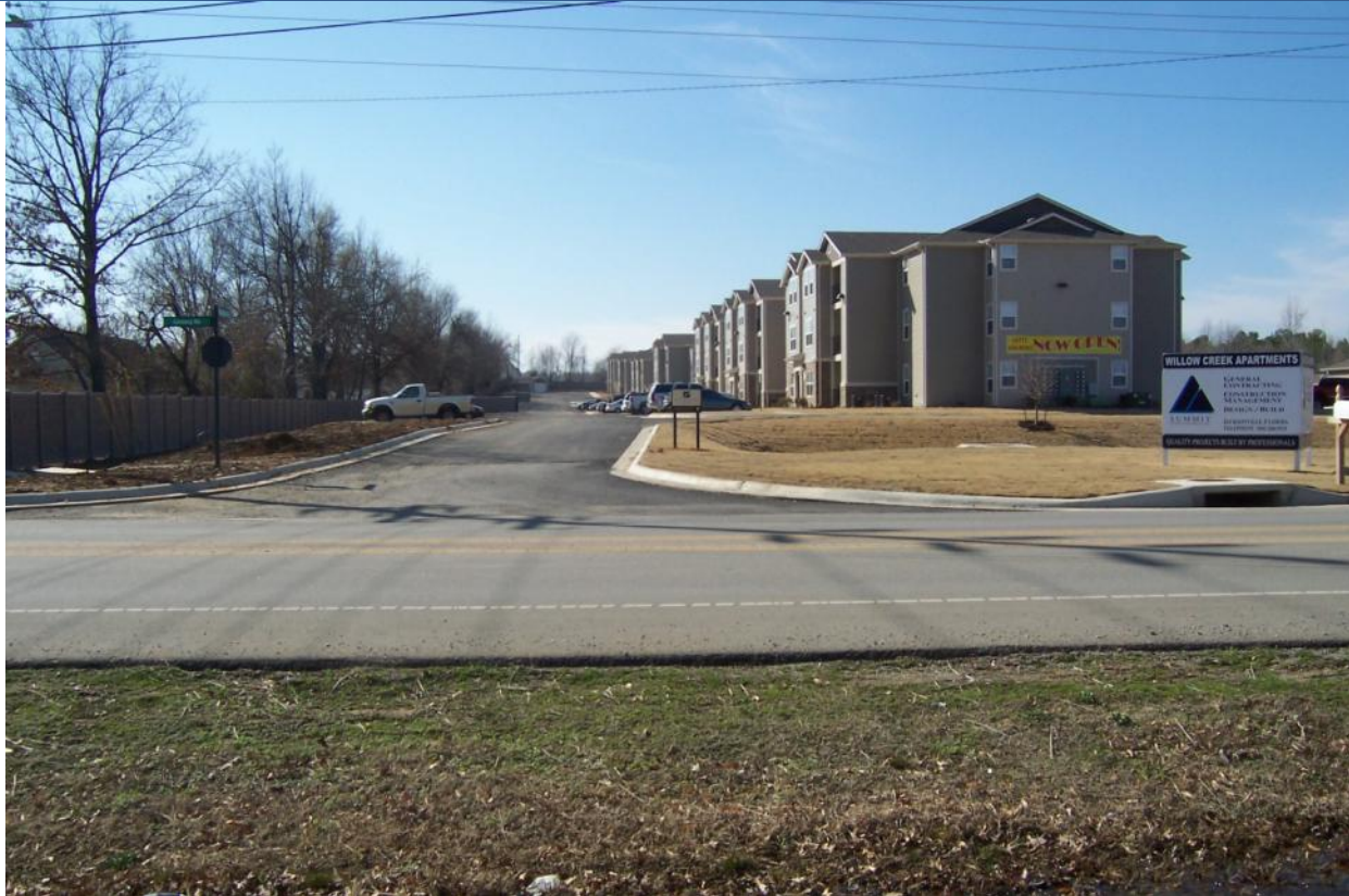
View looking West of apartment entrance (south).
