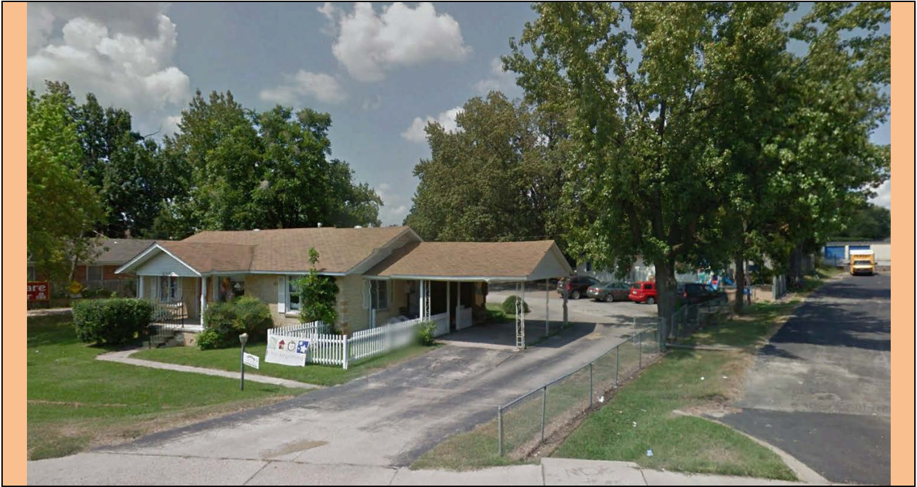
View looking North
