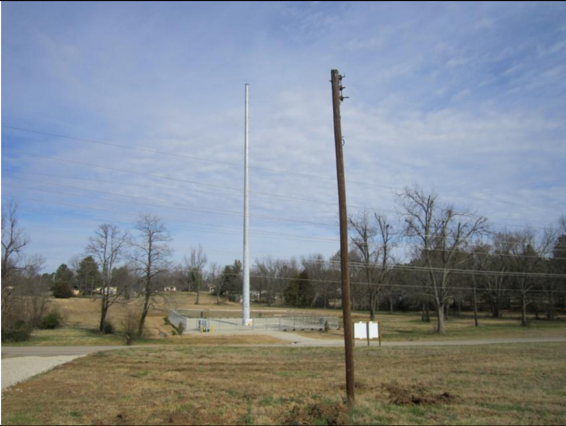
View looking North of the telecommunications tower adjacent from project site.
