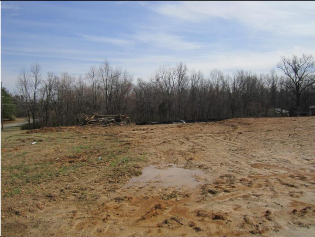
View looking East of proposed church's site.
