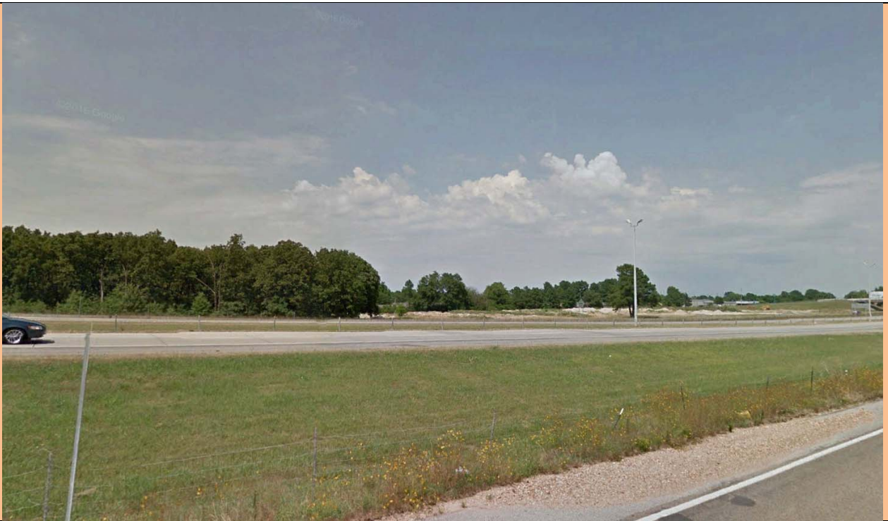
View looking North
