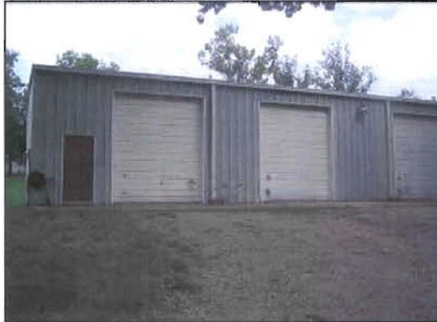
View looking North at subject building
