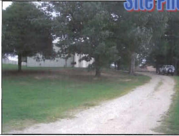
View looking East at subject building
