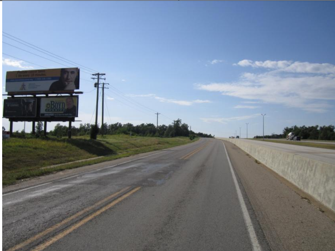
View looking Northwest along Parker Rd. Frontage & I-63
