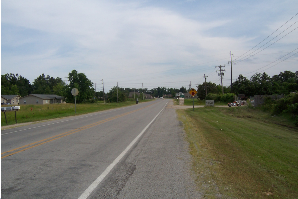
View looking South towards Harrisburg Rd.
