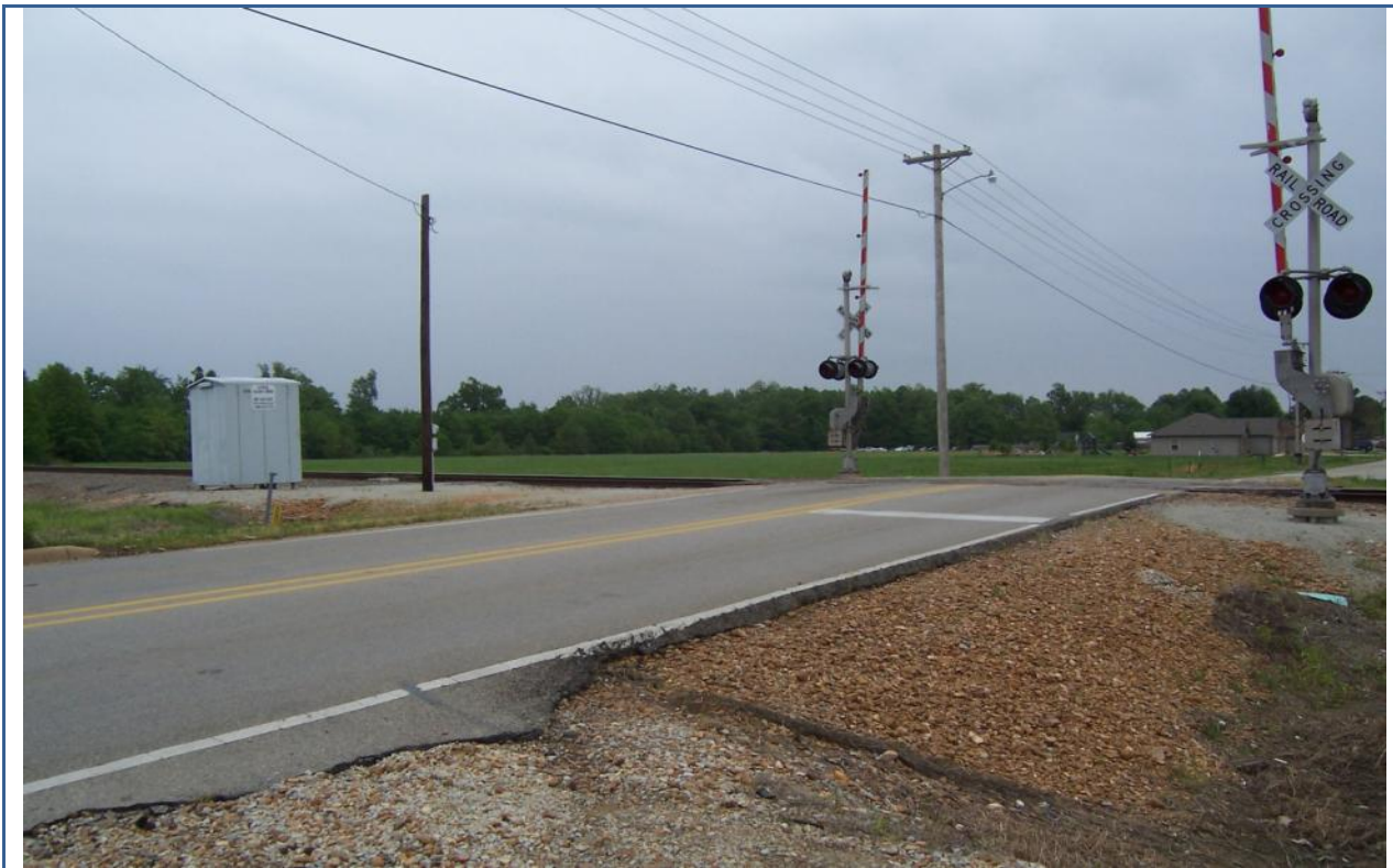
View looking Northeast towards site
